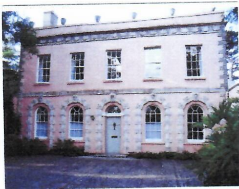
Home of Eleanor Coade, Belmont House, in Lyme Regis, Dorset, with Coade stone ornamental facade
